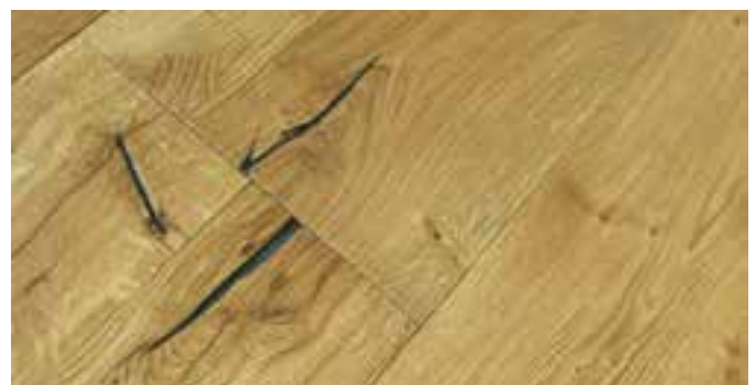
Detail: Cracks Eiche Windsor
